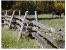
are notched into the logs an inch or so to prevent rolling. Gravity is employed to create vertical stability and lastly 2 pickets are wired across the end of each section to provide lateral stability. The traditional length of each section is a rod (16.5 feet)
