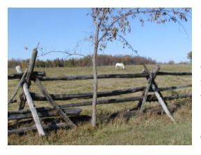
Newer fences on this property are patent fences. A popular fence, it can be seen on many properties in Lanark County. This fence is built above ground with no post holes required and still has excellent lateral and vertical stability. There are many variations of patents, but the idea of the patentee was that they would collect a fee from you for using the design. The patent has long since expired.
